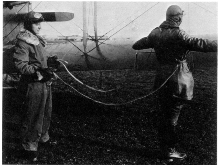
An observer and pilot demonstrate steering the pilot to the objective by reins.
